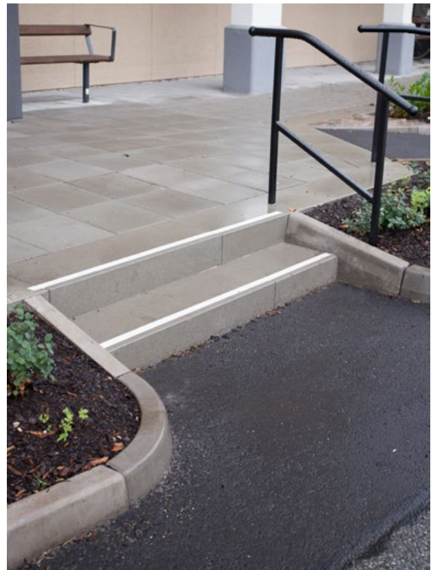
BENDER SPIKMA STREET KERB AND BENDER STAIR BLOCKS
